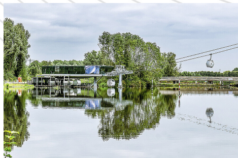
PASSENGER AND MATERIAL TRANSPORT
