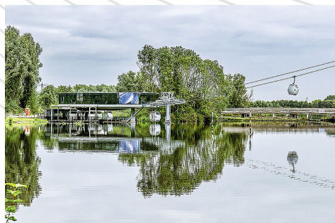
PASSENGER AND MATERIAL TRANSPORT
